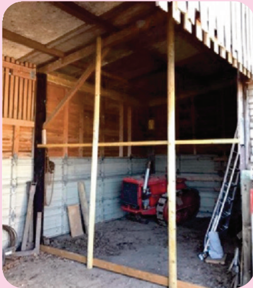
New barn enclosure
